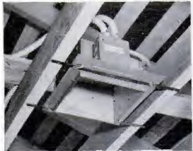
Pyrene & Co., Pomona, Calif., photo Top, even the inside of the lens on this flush light can be cleaned without removing the fixture frame. Mounting strips on lights make installation easy
